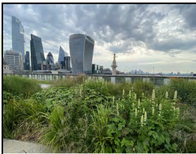
Intensive green roof - London.
